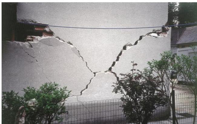
Figure 2: Typical damage caused to houses in the town of Bovec during the 1998 earthquake (photo: Matija Zorn).
