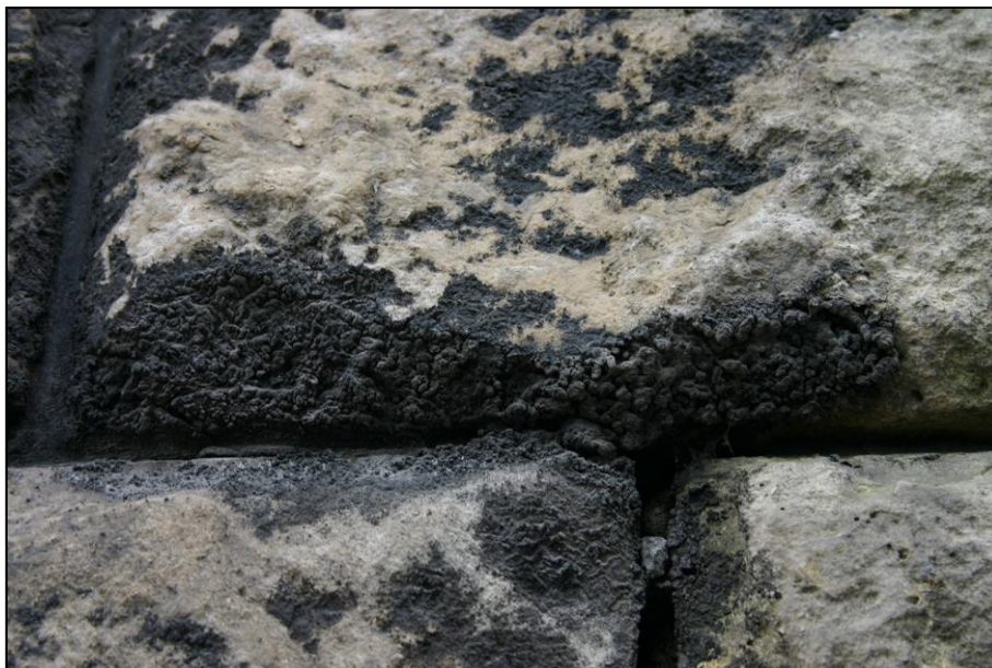
Figure 1. Black gypsum-rich crust.
