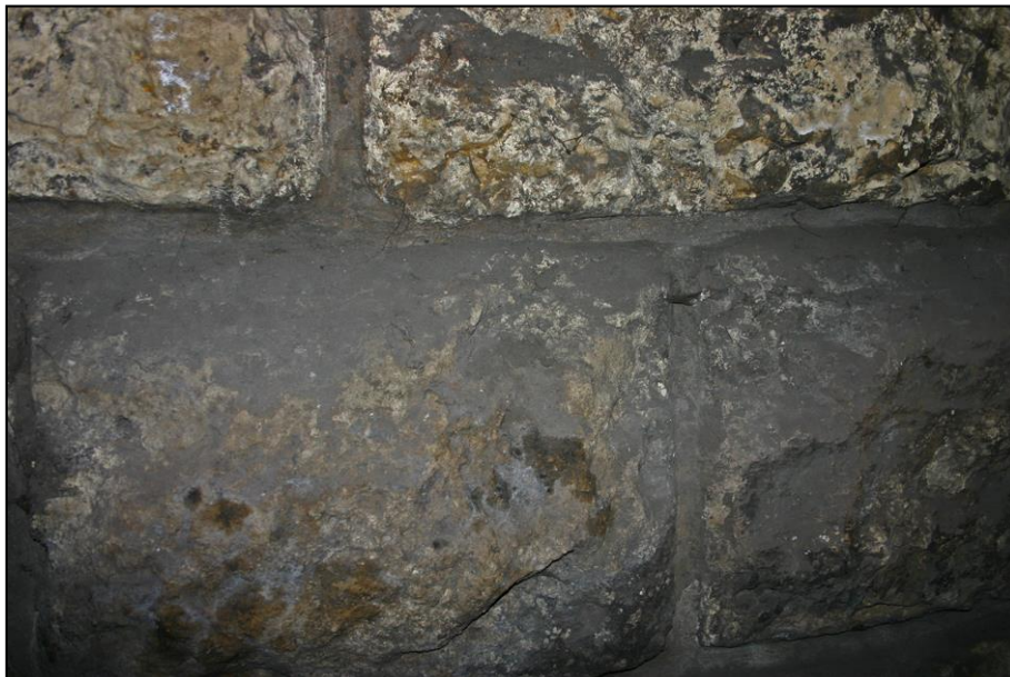
Figure 3. Dark grey crust on the surface of sheltered walls.
