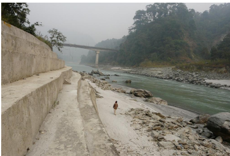
Photo 1. Reinforcement and reprofiling of the Teesta channel banks (Teesta Bazaar)
