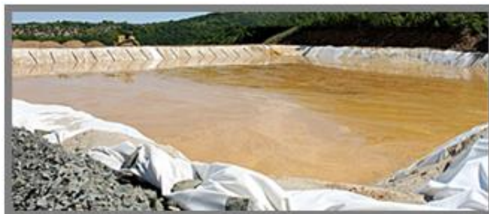
Figure 6. “Ada Tepe” gold mine deposit, integrated mine waste facility (IMWF) – South valley sump
