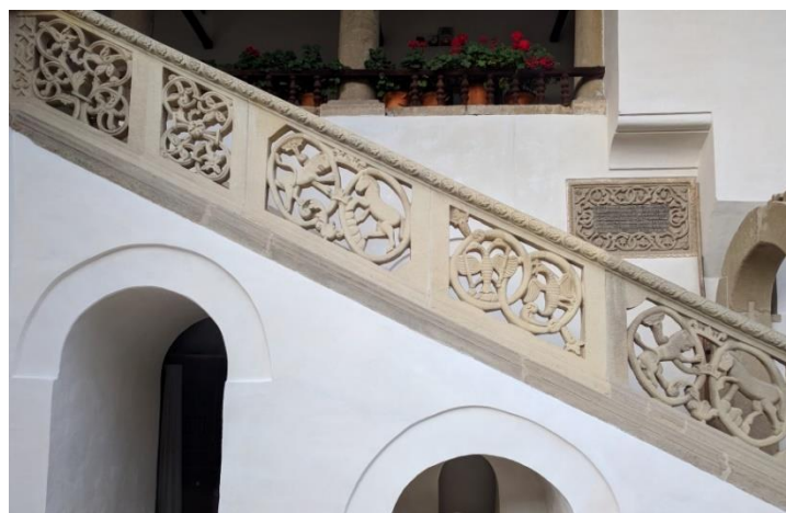
Figure 7. The bannister of the access stairs to the oriel/ watch-tower of Dionisie Bălăcescu
