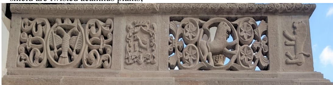
Figure 5. The bannister on the left side of Dionisie's oriel/ watch-tower
