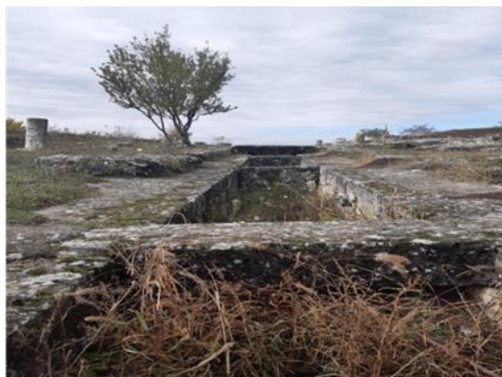
Figure 3. The Tropaeum Traiani citadel-the sewer system alongside the main road
