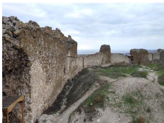
Figure 10. The Enisala Citadel – inner view of the wall
